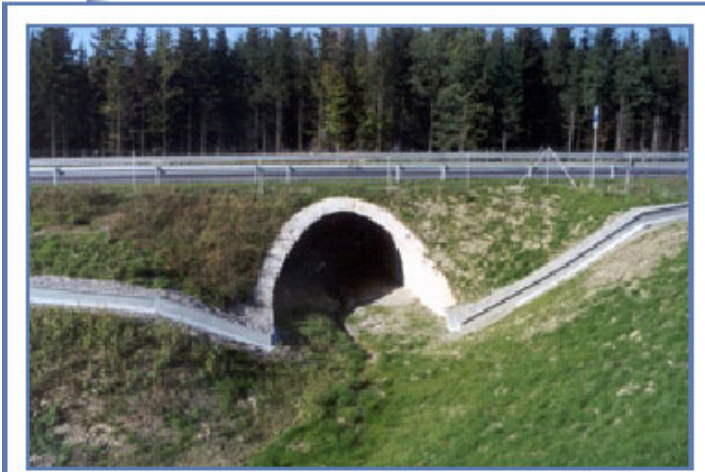
Figure 14. Arch culvert on German Highway B-30, with rail for amphibians and fence for larger wildlife.
