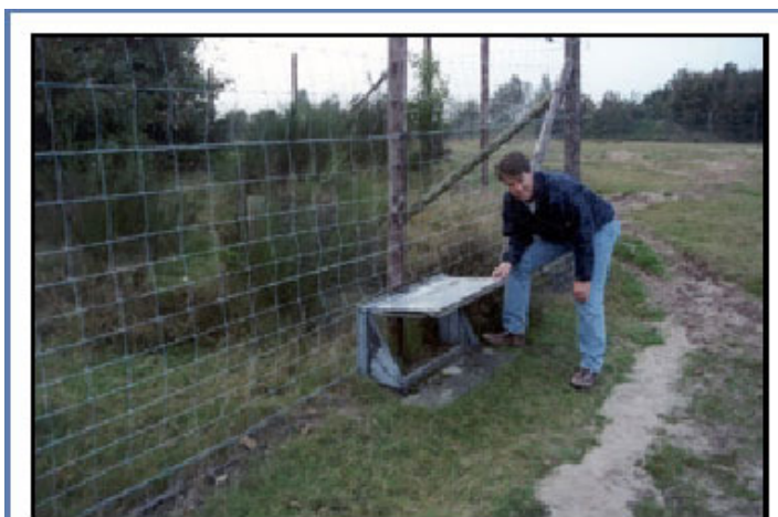
Figure 8. One-way door for small mammals on fence near
