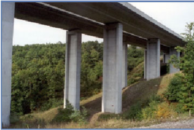
Figure 21. Slovenian viaduct built for wildlife, hydrology, and human connectivity.
