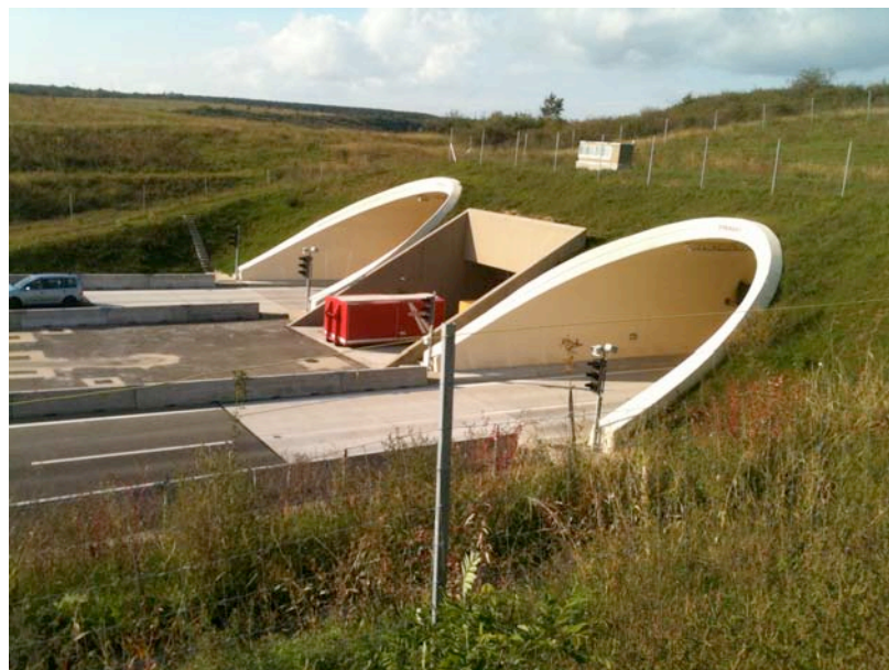
Figure 6.1. Entrance to tunnel in southern Hungary on M7 motorway. The tunnel is under moderately sized hill in agricultural landscape which also supports numerous roe deer
