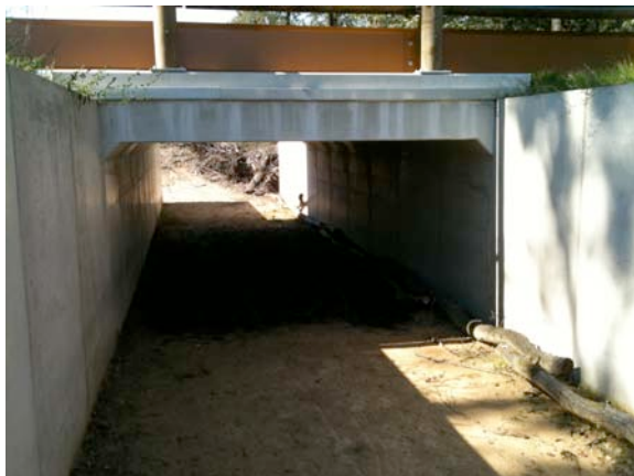
Figure 7.5. Floor of recently constructed box culvert underpass showing sand/earth surface and habitat logs (The Netherlands)
