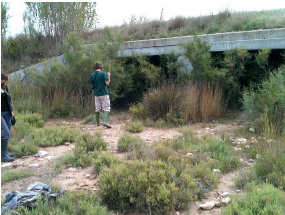
Figure 7.3. Entrance to large multiple box-culvert underpass in Parc Natural deis Aiguamolls de l'Empordia, Cosa Brava, eastern Catalonia, Spain. This underpass is used daily by large numbers of wild boar, as well as numerous other local mammal species. Although the floor of the culvert was originally concrete, this has now been covered in silt. Although no plants grow inside, the natural vegetation on either end is continuous with the surrounding habitat.
