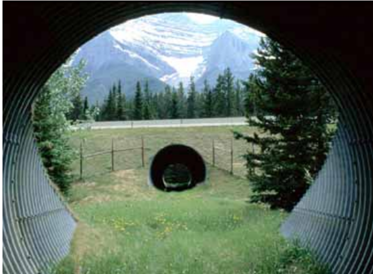
Figure ES15. Photo. Large culvert with vegetative cover and fencing on Highway 1 in Canada (copyright: Tony Clevenger).
