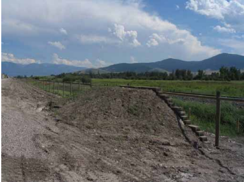
Figure 48. Photo. Jump-out or escape ramp along U.S. Highway 93 on the Flathead Indian Reservation, MT (copyright: Marcel Huijser, WTI).
