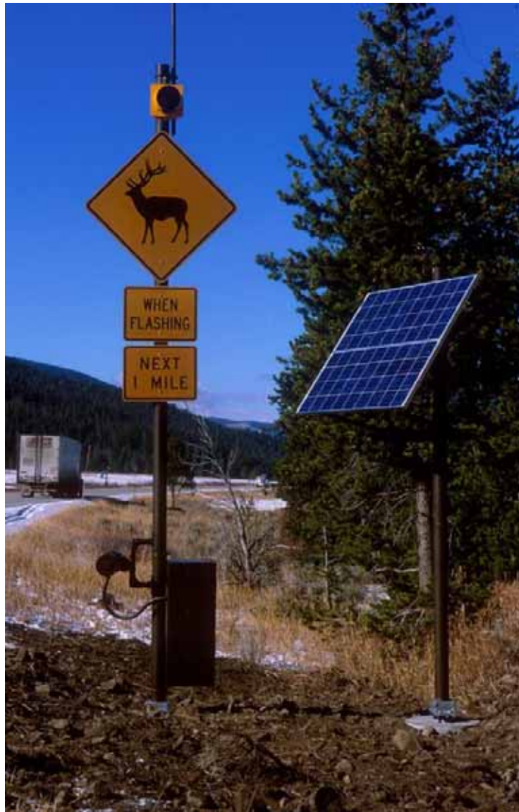
Figure 38. Photo. Animal detection system along Highway 191 in Yellowstone National Park, MT (copyright: Marcel Huijser, WTI).
