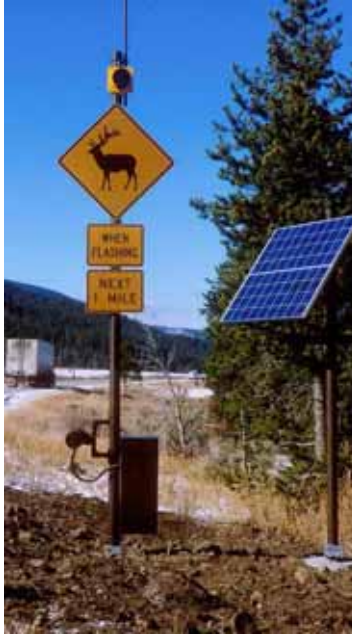
Figure ES19. Photo. Animal detection system along U.S. Highway 191 in Yellowstone National Park, MT (copyright: Marcel Huijser).
