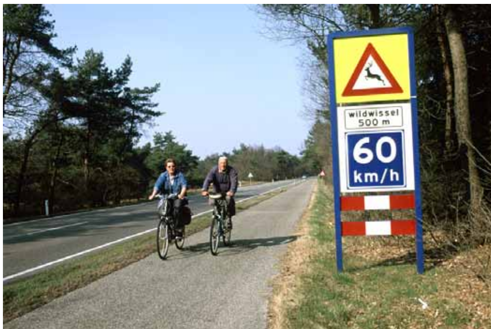
Figure 39. Photo. Advisory speed sign in The Netherlands located at a gap in exclusionary wildlife fencing (copyright: Marcel Huijser).
