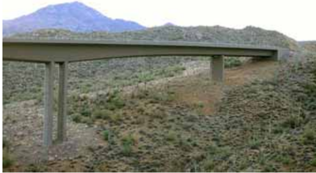
Figure ES16. Photo. Long bridge on Arizona Highway 260 constructed in such a way as to minimize the impact to soil and vegetation (copyright: Marcel Huijser).
