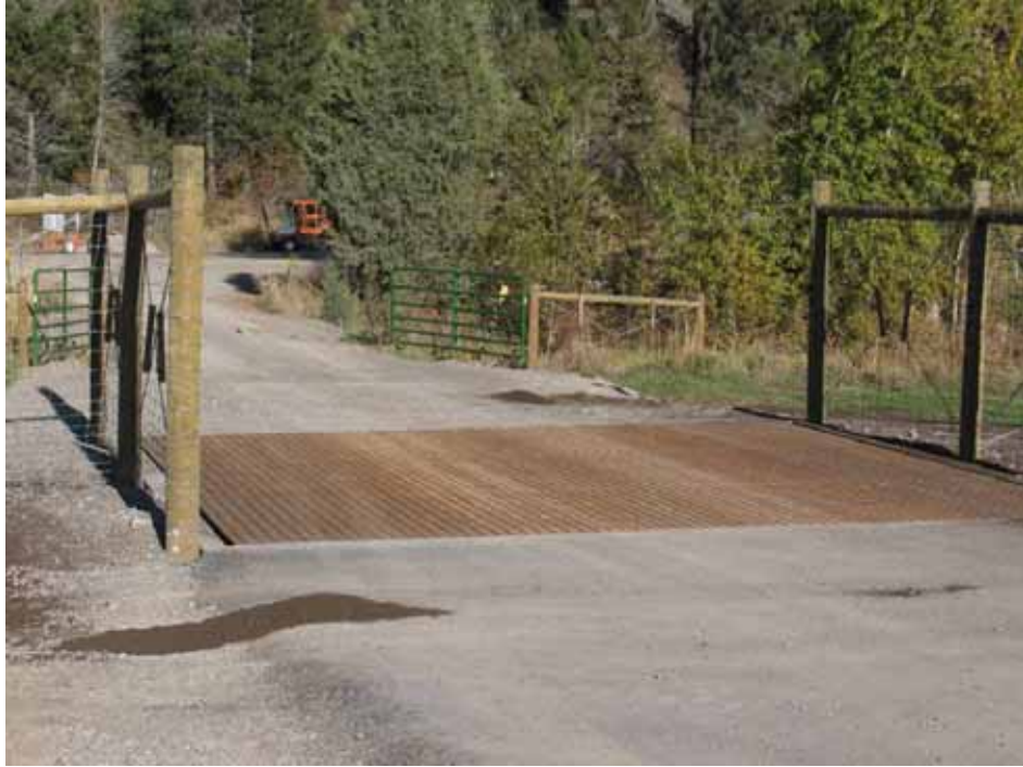
Figure 52. Photo. Wildlife guard along U.S. Highway 93 on the Flathead Indian Reservation, MT (copyright: Marcel Huijser, WTI).
