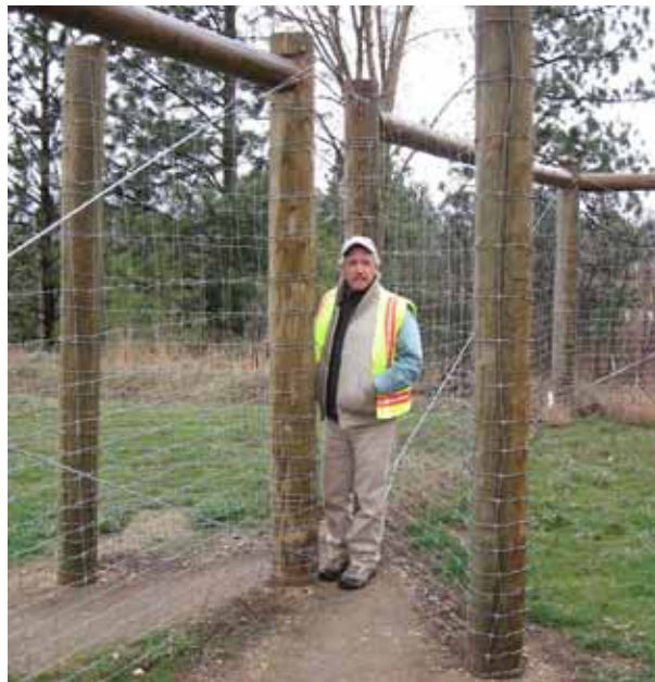
Figure 53. Photo. Angled opening in fence allowing access for people along U.S. Highway 93, MT (copyright: Marcel Huijser, WTI).
