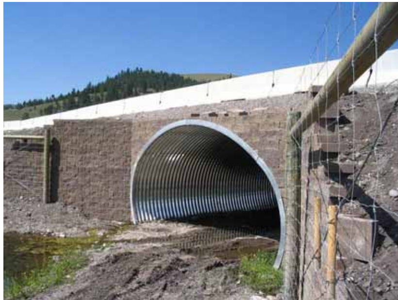
Figure 45. Photo. Wildlife underpass along U.S. Highway 93 on the Flathead Indian Reservation, MT (copyright: Marcel Huijser, WTI).
