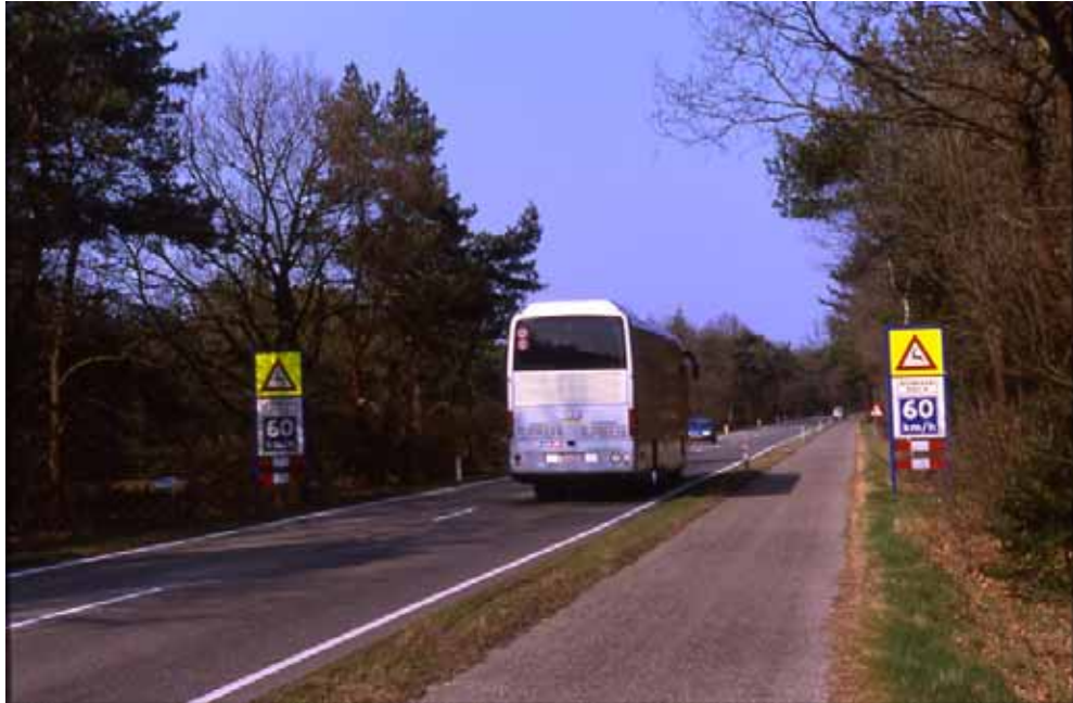
Figure 43. Photo. Gap in a wildlife fence accompanied by wildlife warning signs and advisory speed limit reduction, The Netherlands (copyright: Marcel Huijser).
