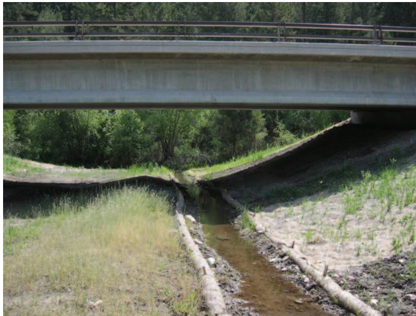
Figure 58. Photo. Long bridges do not have to be excessively large to provide ample space for wildlife crossings. While not exceedingly long, this bridge provides plentiful space for both the stream and wildlife to cross.
