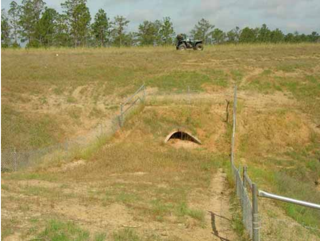
Figure 23. Photo. Fences lead gopher tortoises towards a culvert along Highway 63 in Green County, south of Leakesville, MS (copyright: Chuck Walters, Environmental Division, Mississippi Department of Transportation).
