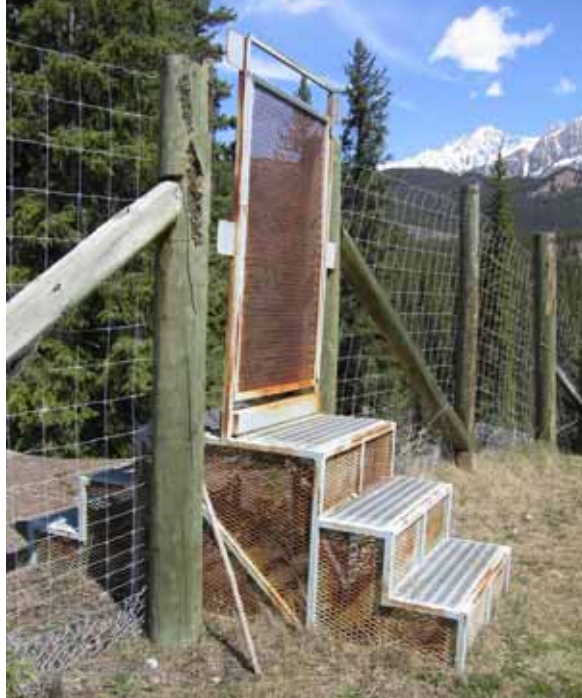
Figure 54. Photo. Swing gate in fence (spring loaded) allowing access for people, along the Trans-Canada Highway in Banff National Park, Alberta, Canada (copyright: Adam Ford, TCH research project/WTI-MSU).
