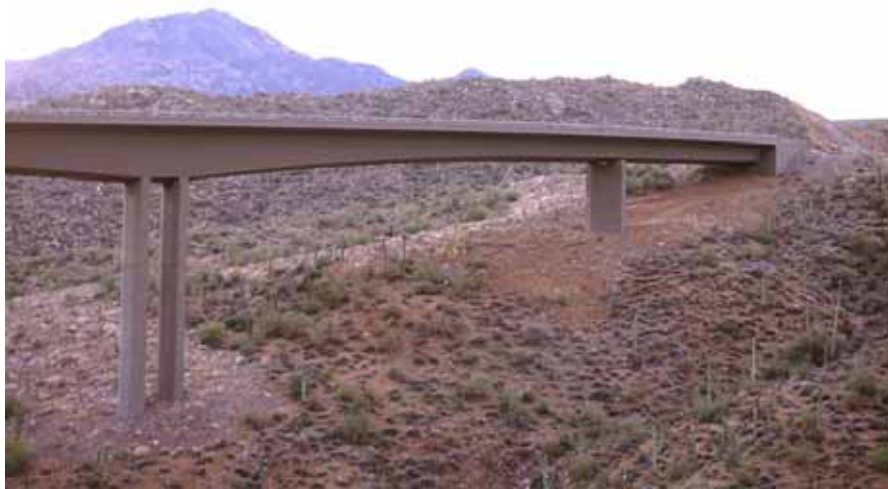
Figure 57. Photo. Long bridge on Arizona State Route 260 constructed in such a way as to minimize the impact to soil and vegetation (copyright: Marcel Huijser).
