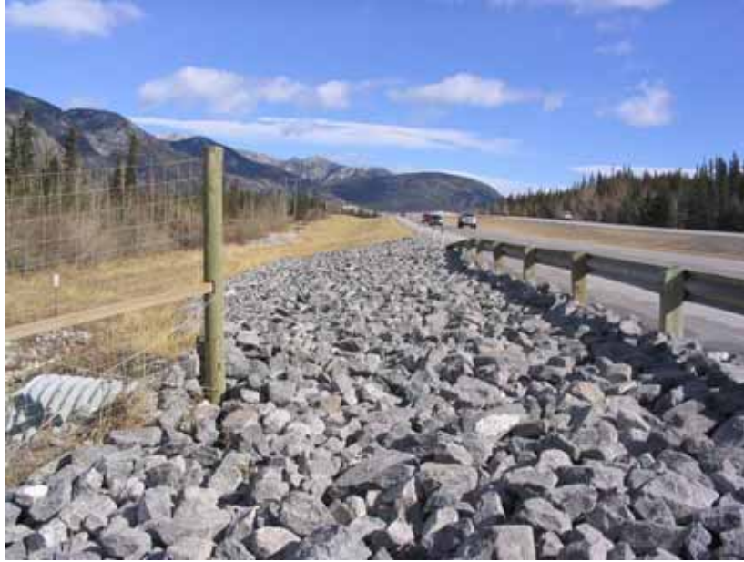
Figure 51. Photo. The boulder field at the fence end at Dead Man’s Flats along the Trans-Canada Highway east of Canmore, Alberta, Canada (copyright: Bruce Leeson).
