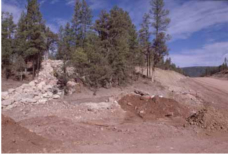
Figure 56. Photo. Large boulders placed in the right of way as a barrier to elk and deer with a view of State Route 260 (under construction) in Arizona (copyright: Marcel Huijser).
