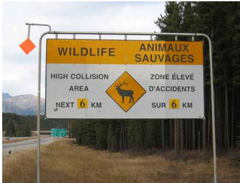
Figure 36. Photo. Large enhanced elk warning sign along the Trans-Canada Highway in Banff National Park, Canada (copyright: Marcel Huijser, WTI).
