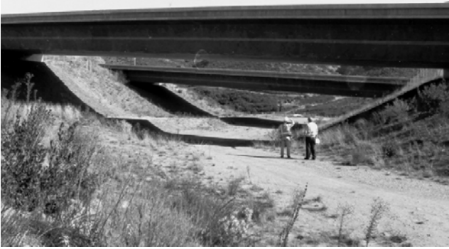
FIGURE 12 Wildlife underpass on Highway 241 in southern California.
