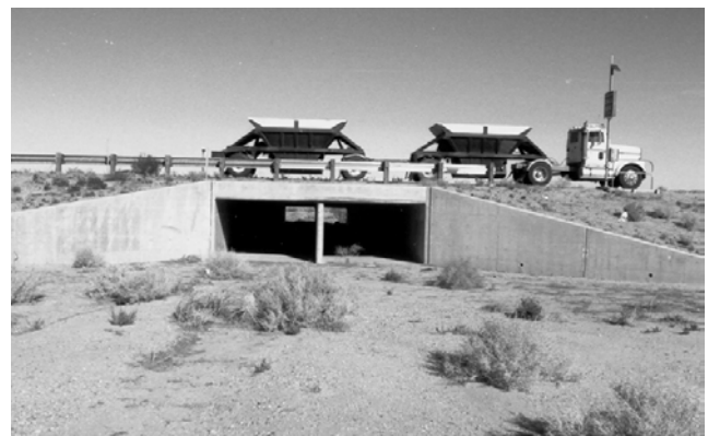
FIGURE 7 Box culvert used by desert tortoise along Highway 58 in California.
