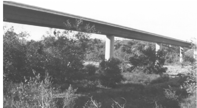
FIGURE 19 Viaduct on Highway 241 in southern California.
