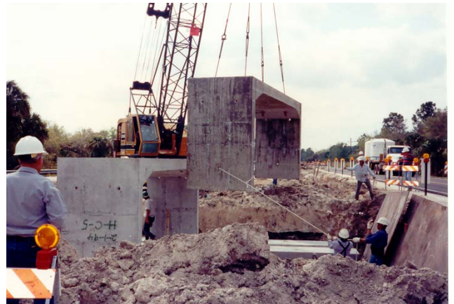
FIGURE 17 Pre-cast segment construction of box culvert wildlife underpass in Florida.
