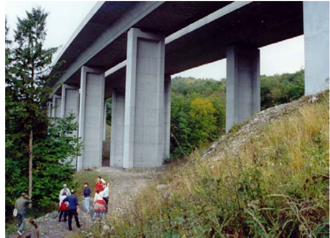
FIGURE 18 Viaduct on the Ljubljana–Trieste Highway in Slovenia.
