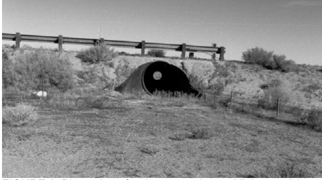
FIGURE 8 Pipe culvert for desert tortoise on Highway 58 in California.
