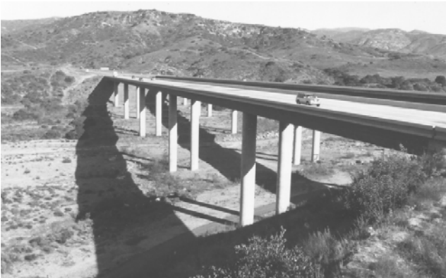
FIGURE 13 Viaduct on Highway 241 in southern California.
