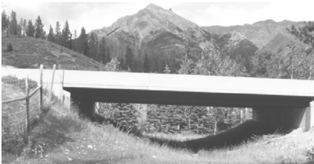
FIGURE 26 Underpass in Banff National Park, Alberta.
