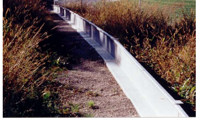
FIGURE 3 Galvanized steel barrier with lip used for reptiles and amphibians in Europe.
