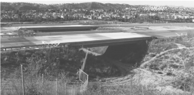
FIGURE 14 California structures suitable for wildlife use but precluded by adjacent development.
