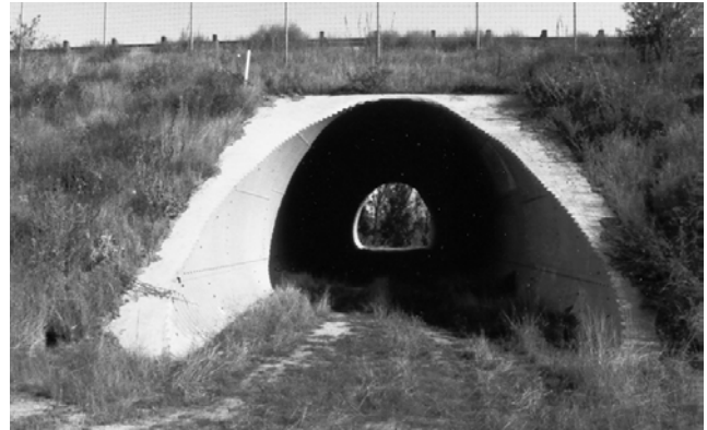
FIGURE 15 Large pipe culvert being used by wildlife under Highway 71 in southern California.
