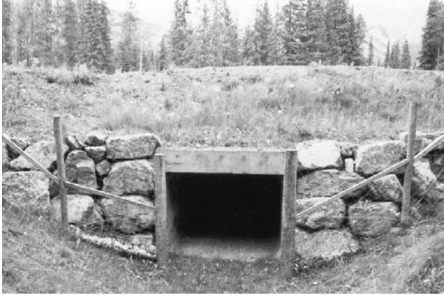
FIGURE 5 Box culvert being used by wildlife in Banff National Park.
