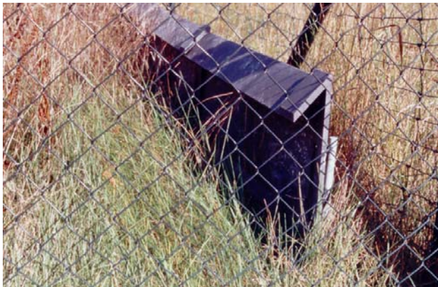
FIGURE 2 Plastic barrier with angled lip used for reptiles and amphibians in Europe.
