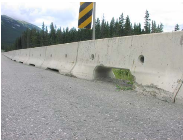
Figure 40: Concrete barriers with scuppers for small to mid-sized animal passage. Photo by A. P. Clevenger.
