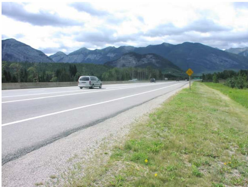
Figure 38: Solid concrete barriers often stretch continuously for miles. Photo by A.P. Clevenger.
