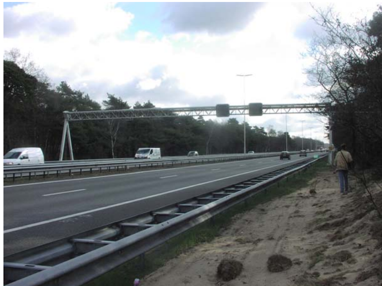
Figure 42: Doubled metal beam median barrier and guardrail. Photo by A.P. Clevenger.
