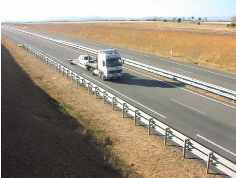
Figure 41: Metal beam barrier and guardrail. Photo by A. P. Clevenger.
