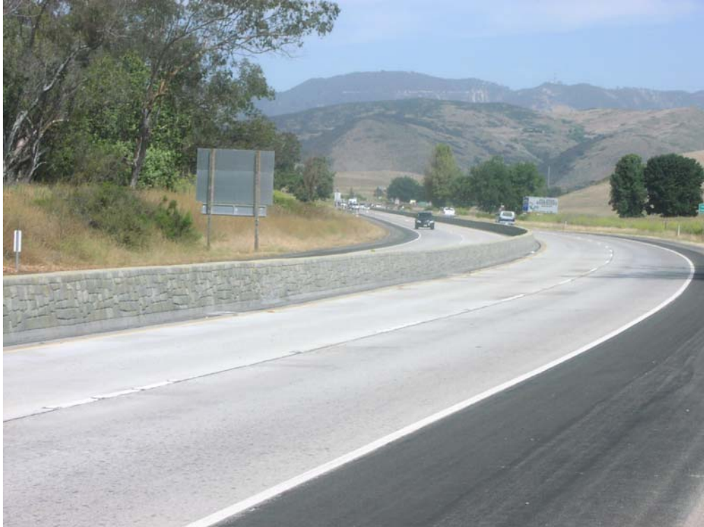
Figure 2: No standards currently exist for spacing of basal openings. Small mammals would be challenged to find passage through this section of median barrier on Highway 1 . Photo by A. P. Clevenger.
