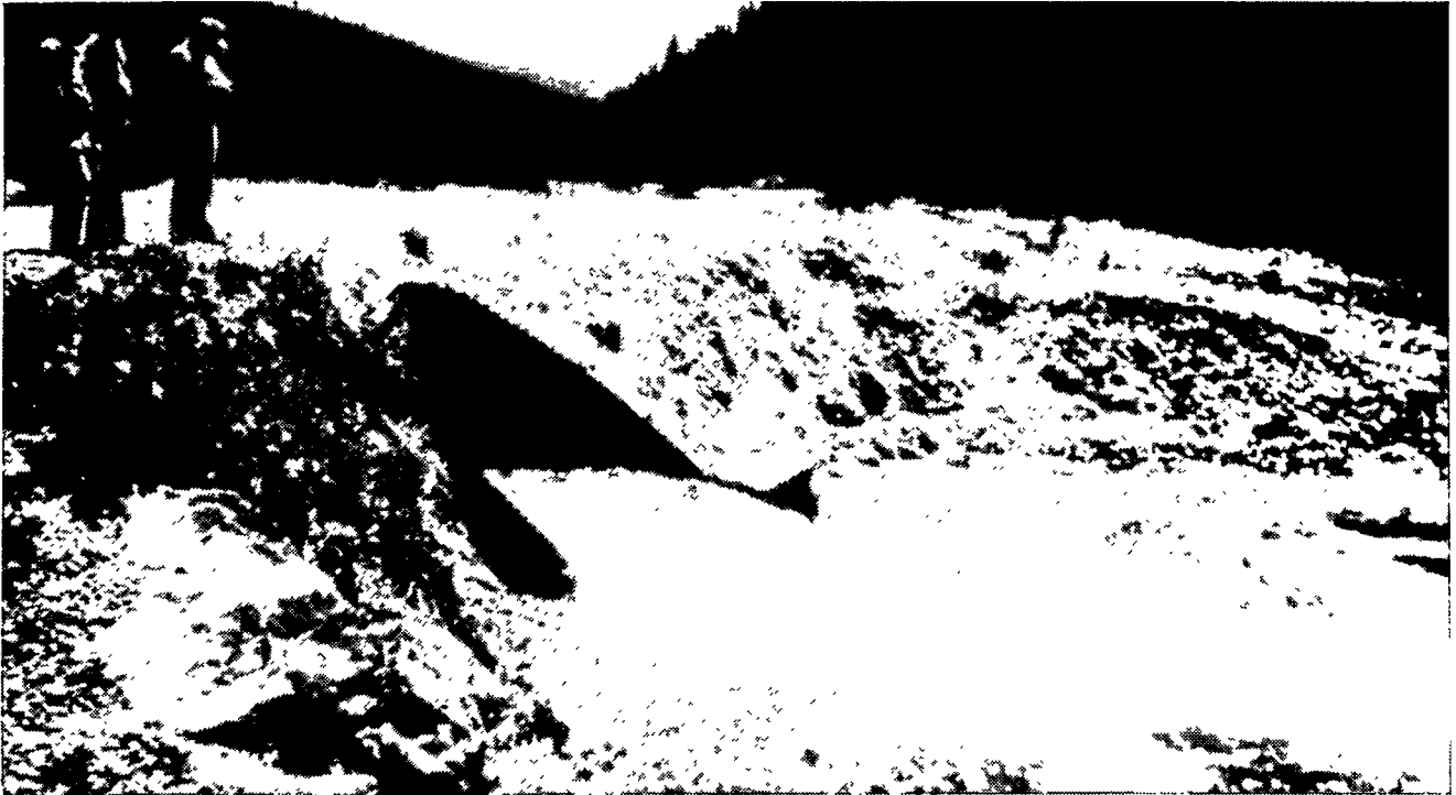
Figure 1. High water velocities and vertical barriers obstruct fish passage
