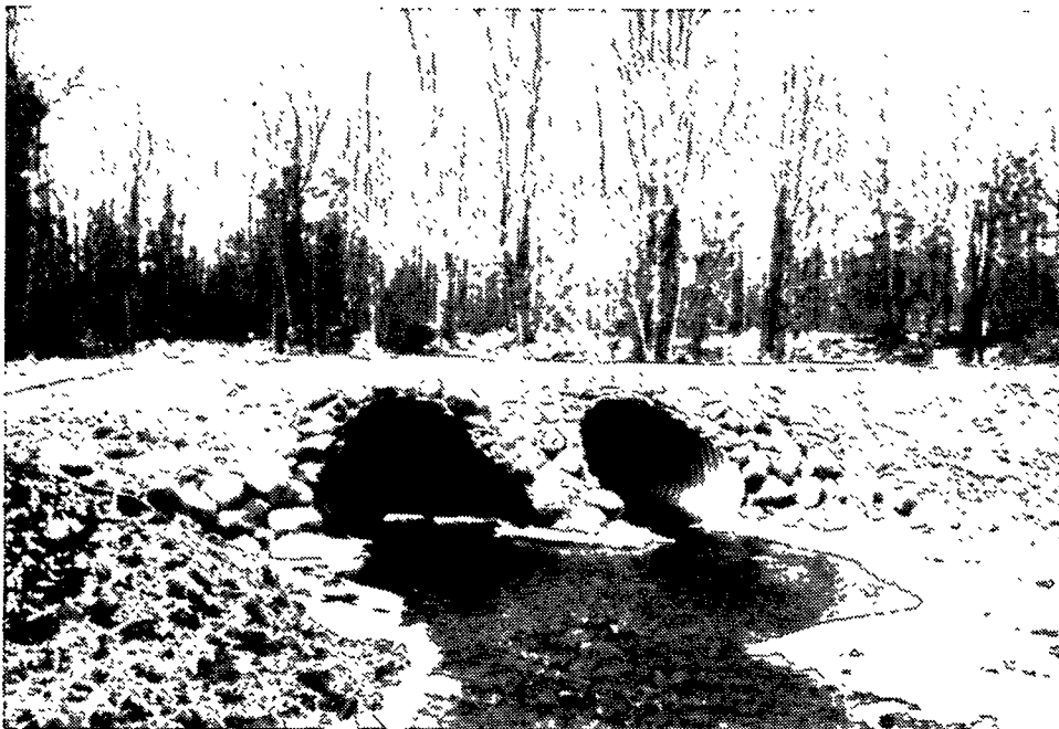
Figure 16. Fish passage may be provided in streams that have wide ranges of flows by providing multiple culverts.
